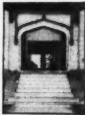
View of Entrance to Main Building
